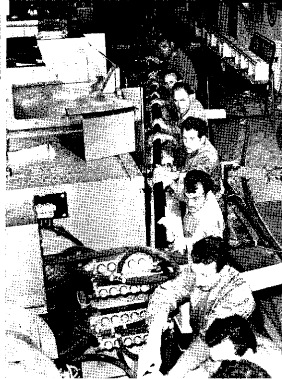
Installation of one of the 'bump coils' added to eight of the PS magnets during the shut-down, in preparation for the planned beam ejection from straight-section 74, intended for neutrino experiments. The coil fits round the yoke of the magnet and the bundle of conductors (here 16 pieces, each of 150 mm 2 cross-section, 11 metres long) had to be eased inside, between the yoke and the screw-jacks separating the main coils, without damaging the insulation of either the new or existing coils.
